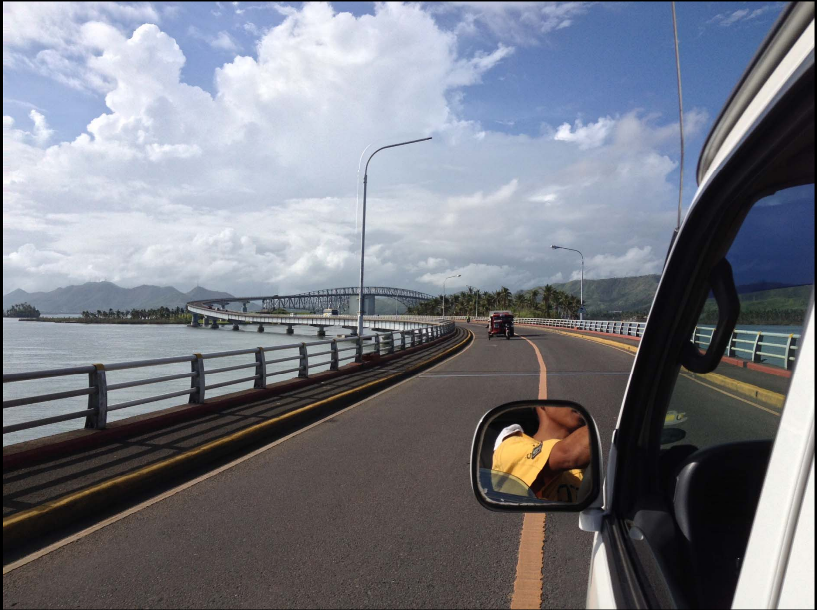
San Juanico Bridge.
