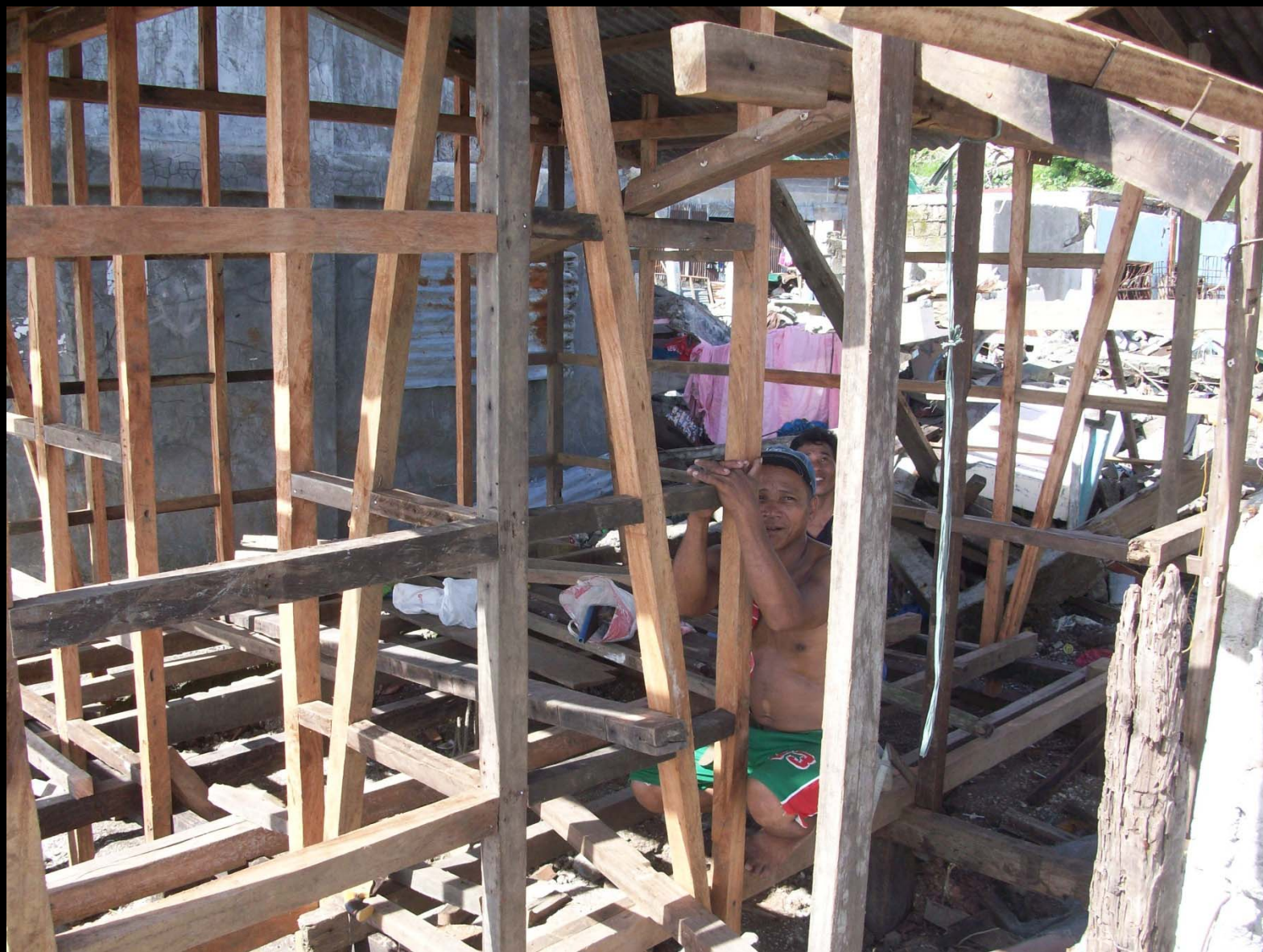
Residents in Basey rebuilding.
