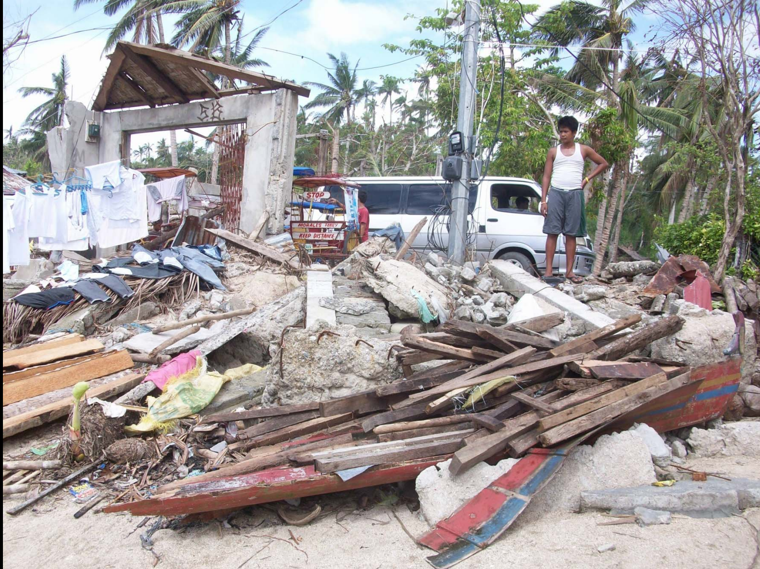
Damage in Barangay San Antonio.
