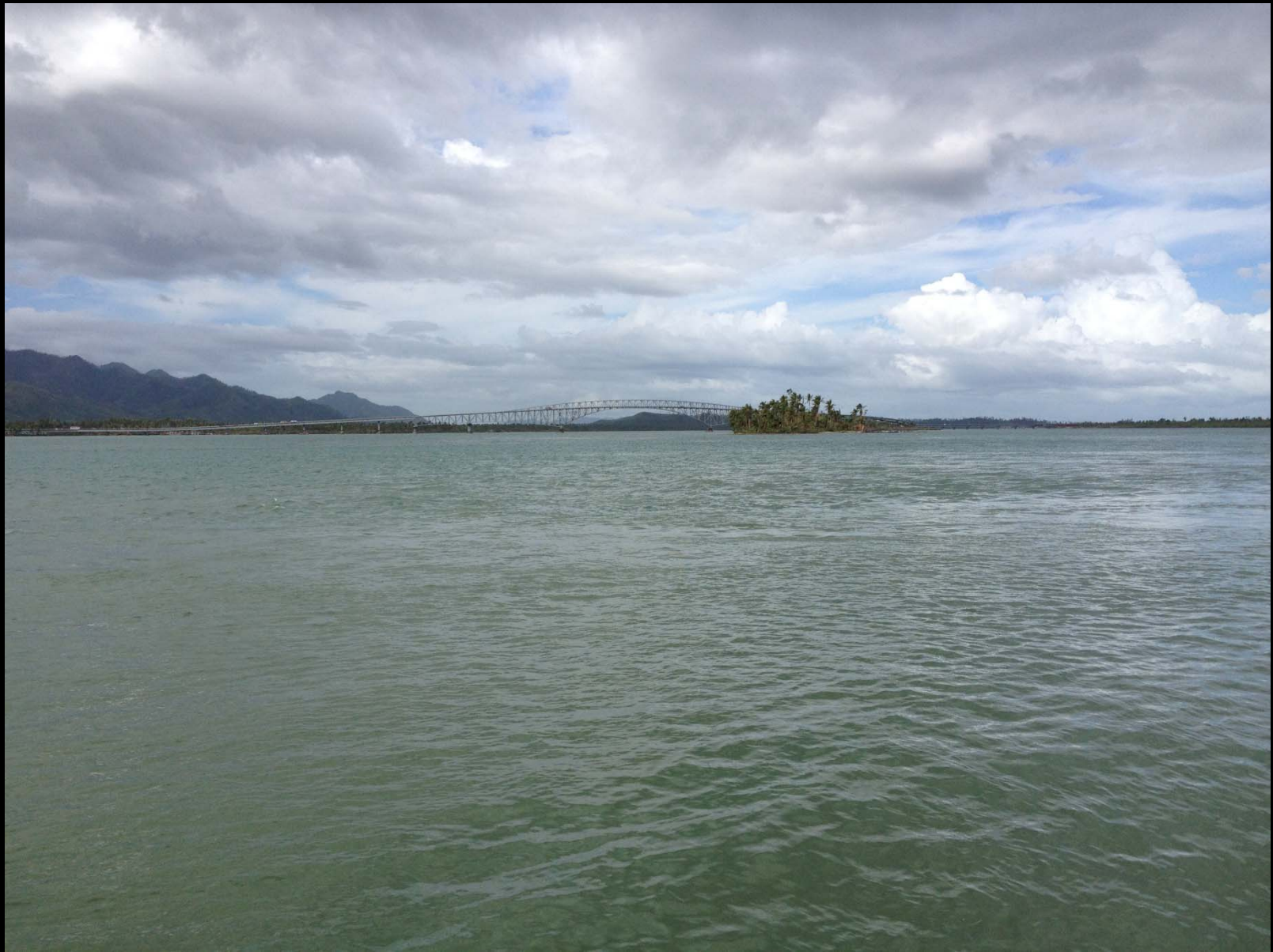
San Juanico Bridge.
