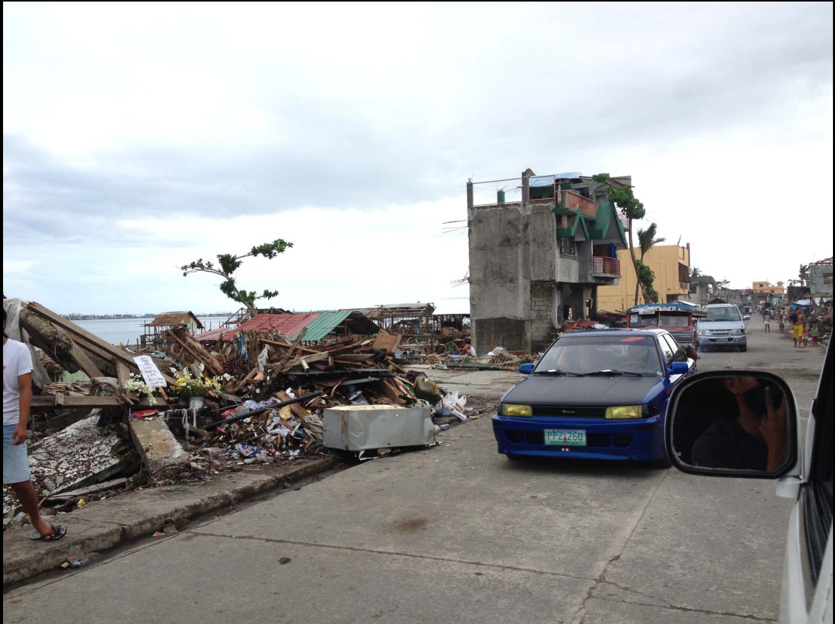
Damage on Tacloban's waterfront.
